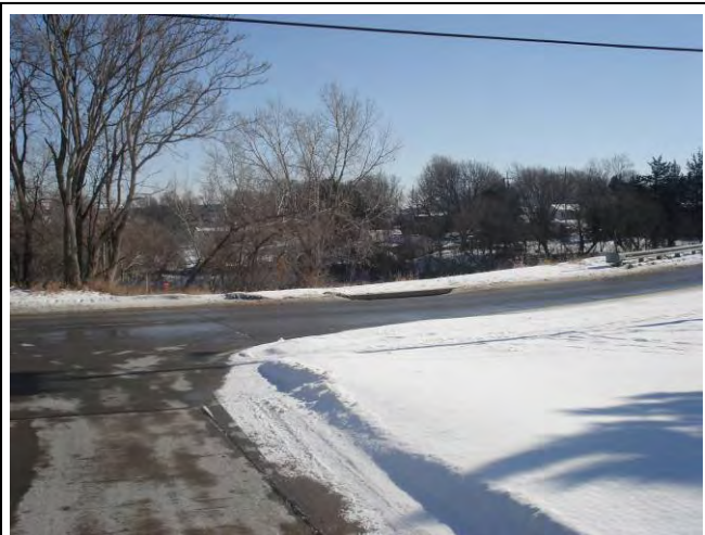
1170 – Looking at street inlet (free of debris)
