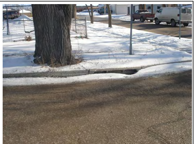
1246 – Inlet on southeast corner of intersection of 20th and U Street
