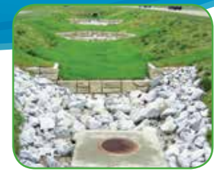
Completed Bioswale System, Florence
