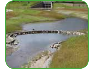
Completed Retention Wetlands, Adams Park
