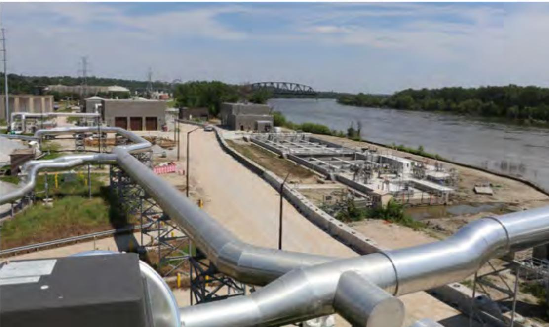
Construction of the Chlorine Contact Basin at the MRWRRF site, looking northeast (July 2019). Note the HESCO flood protection barrier located on the east side of the plant access road to protect treatment facilities from the 2019 Missouri River flooding.
