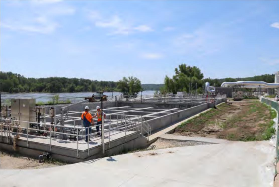
Construction of the Chlorine Contact Basin at the MRWRRF site, looking southeast (July 2019). Taken in-between flood events. HESCO baskets are shown on the right.
