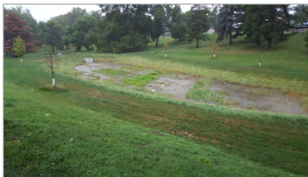
FIGURE 2-17 Hitchcock Park Green Infrastructure
