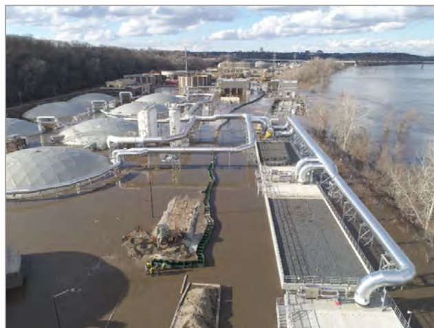
FIGURE 2-32 Flooding at the MRWRRF Site in 2019
