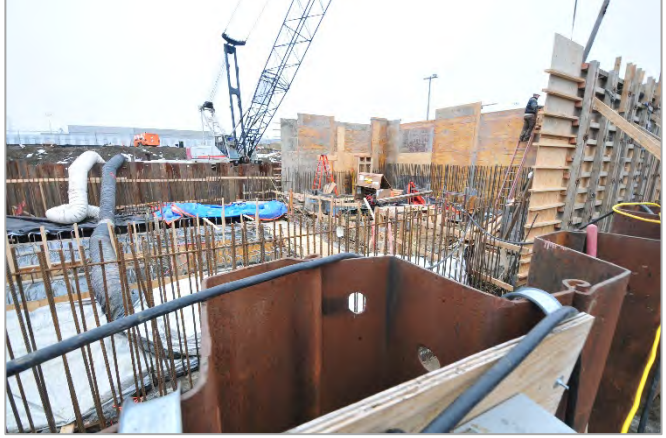
FIGURE 2-9 Riverview Lift Station Under Construction in January 2021 (Courtesy of Multivista)
