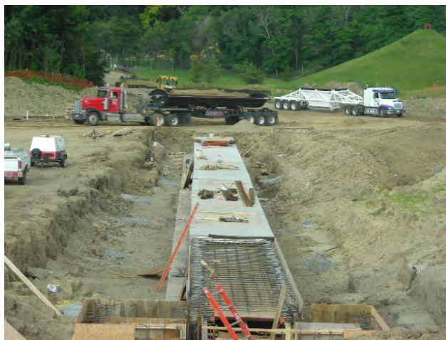
FIGURE 2-8 Construction in Lauritzen Gardens
