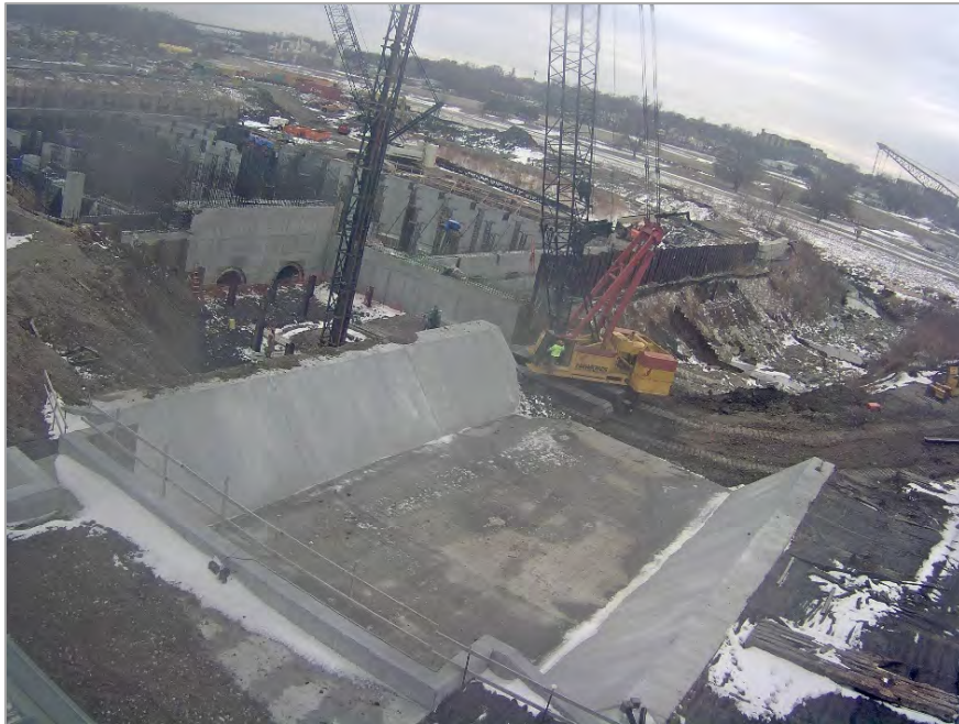
FIGURE 2-16 Construction of the SCRTB January 2021 (Courtesy of Multivista)
