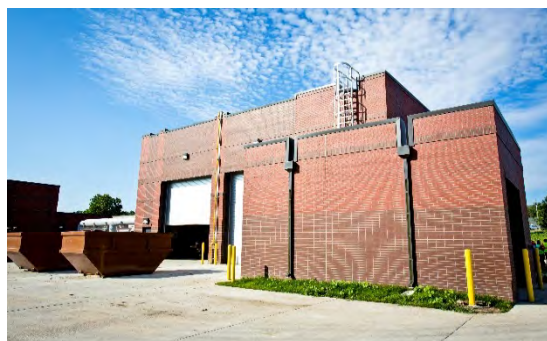
FIGURE 2-11 South Omaha Industrial Area Lift Station
