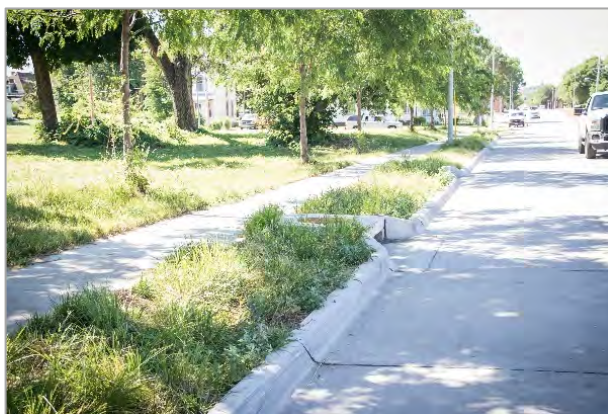
FIGURE 2-6 Curbside Retention Ponds on the 26th and Corby Project
