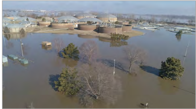
FIGURE 2-33 March 2019 Flooding at PCWRRF
