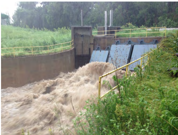
FIGURE 2-2 CSO 105 Minne Lusa Avenue Discharge during a June 2014 Storm
