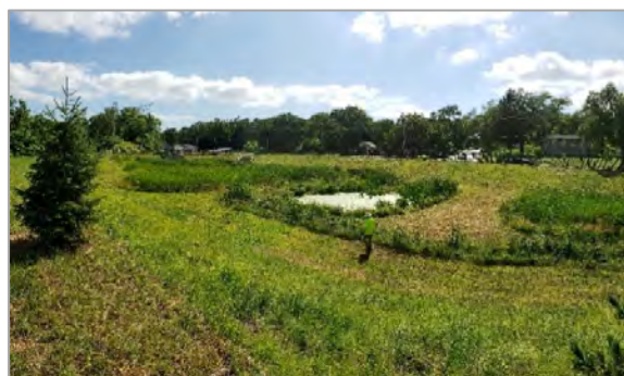
FIGURE 2-12 Gilmore Detention Basin
