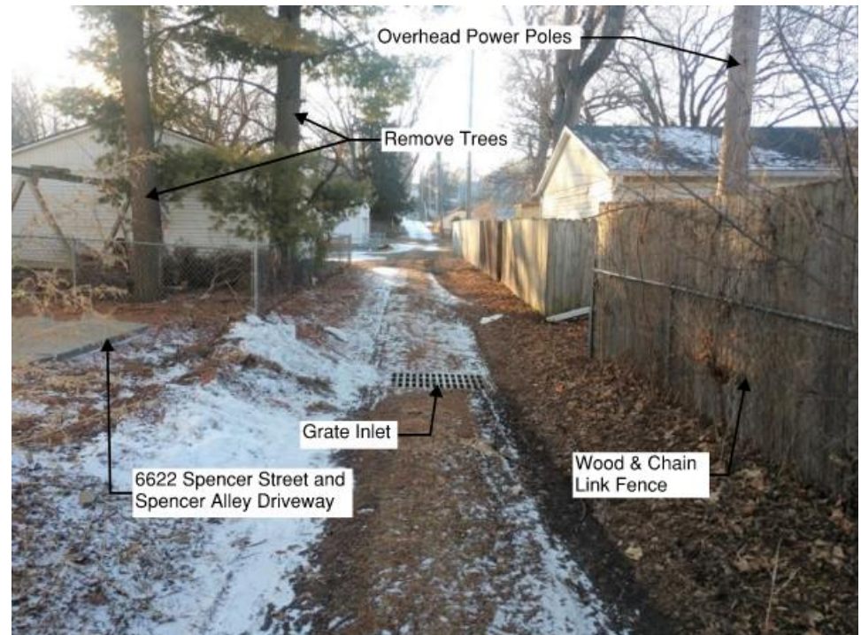
Picture 2 - Looking west to N. 67 th Avenue
