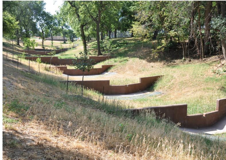
For this project, new storm sewers were extended north and east to approximately 56th and Marcy Streets. Some of the new storm sewers carry stormwater north to Elmwood Park where it flows through a series of detention ponds referred to as the "Elmwood Diversion". These ponds provide a cost effective, green stormwater solution by:
